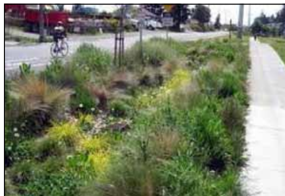
Courtesy photo Vegetated swales in developed areas help to infiltrate water into the ground.
